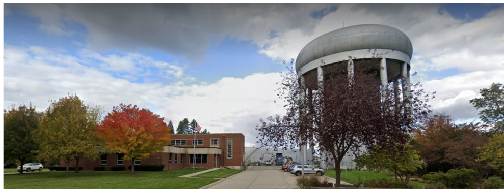
Southeastern Oakland County Water Authority Headquarters Royal Oak Side of Webster Road – North of Pattengill School
